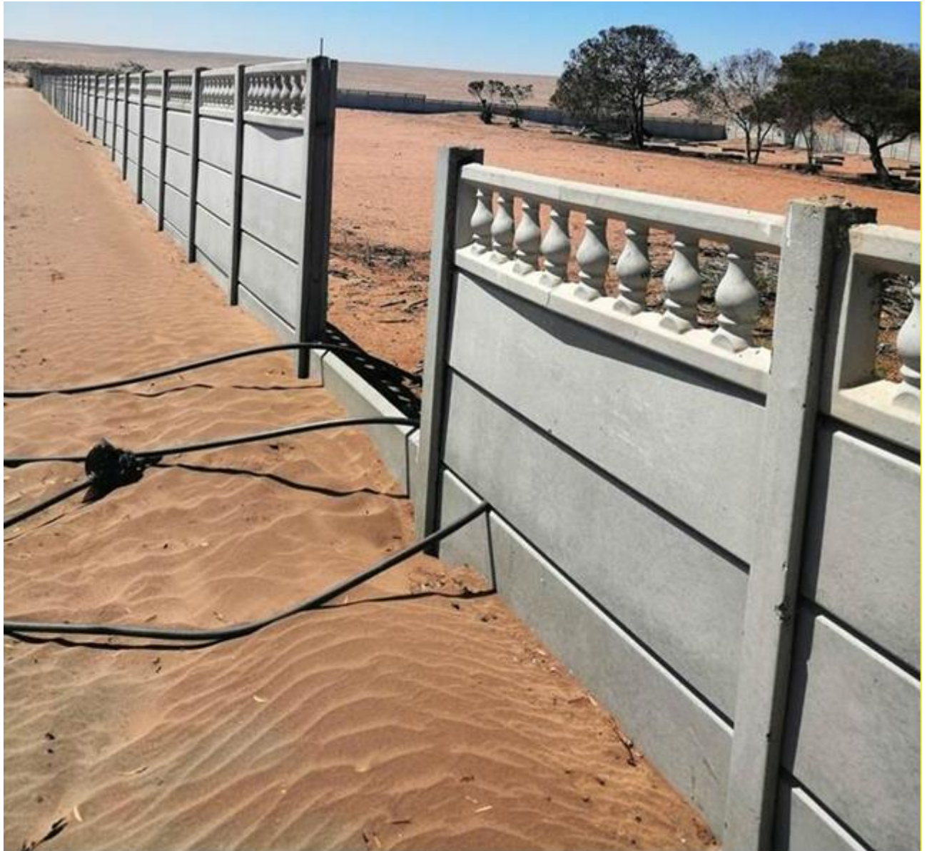
Picture 1 - Boundary Wall to be demolished
